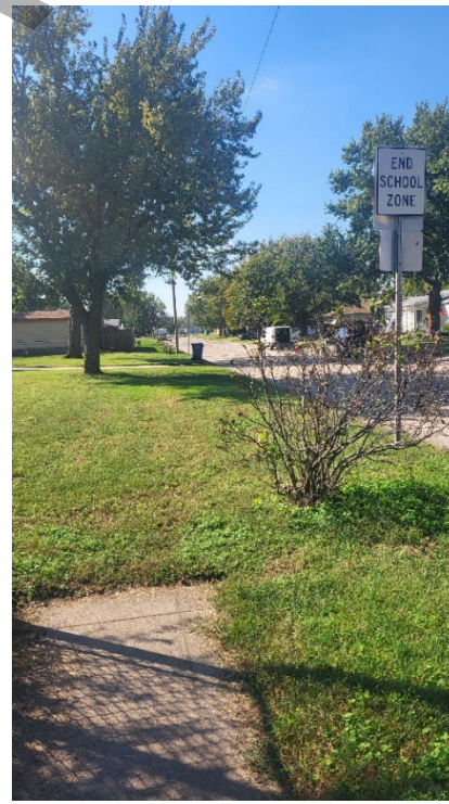
Incomplete sidewalks at St. Anne Catholic School
