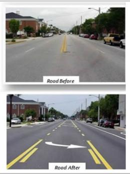
econfiguration known as a road diet offers several highvements at a low cost by reallocating vehicular lanes. The efits of a road diet include enhanced safety, mobility and l road users and a "complete streets" environment to ate a variety of transportation modes. A road diet can better ning vehicles, encourage safer speeds, and potentially add pace for cyclists or transit.
